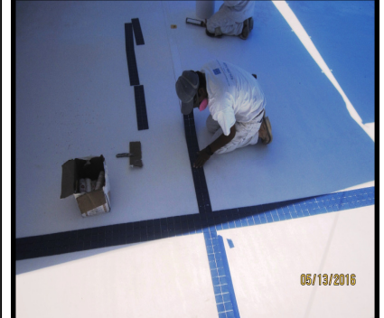
Installing Tile in Bottom
