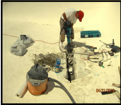
Splitting the Drain
